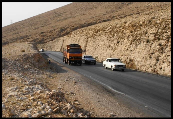
Unsafe overtaking of sedan vehicles due to high traffic of heavy vehicles
